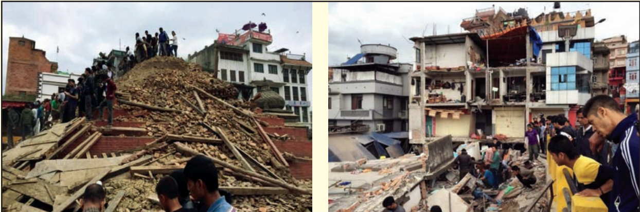
Devastation of Buildings due to Nepal Earthquake
